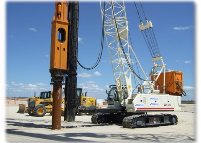
➤ CSP Steel Plant Project, Brazil
