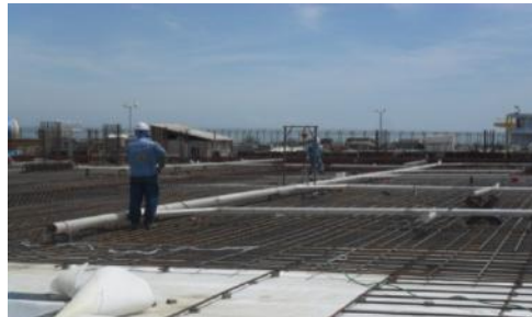
➤ KHNP GORI Contaminated Water Pipeline Replacement Project
