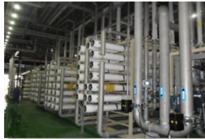
(Industrial Water/Pure Water/RO /UDI System)
