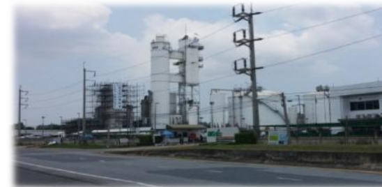
◀ N2 Liquefaction Plant in Thailand♪
