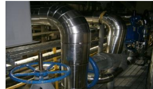
➤ KHNP YOUNGKWANG Heat Exchanger Pipeline Replacement Project
