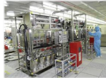
FAB Equipment Hook-Up
