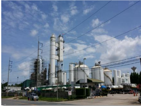
➤ BIG Nitrogen Liquefier Plant ▶ 10
