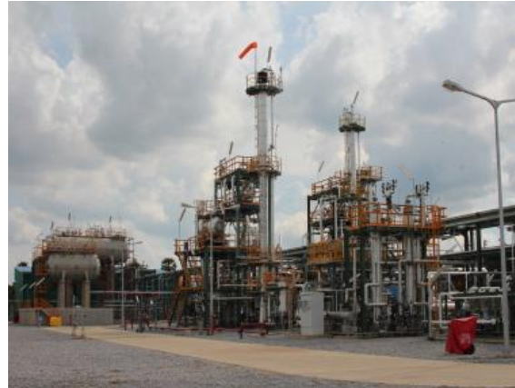
➤ THAI Gas Separation Plant ▶ 13
